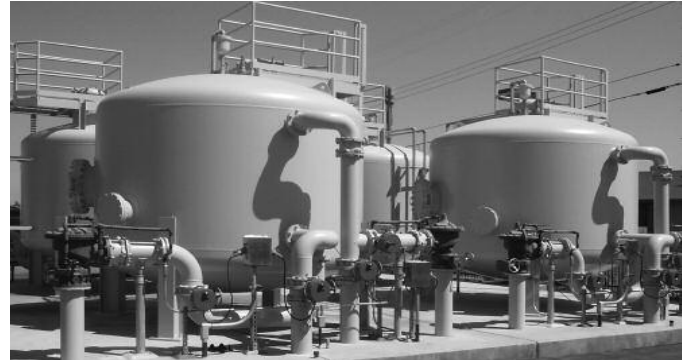
MetalEase-61 Installation in Elk Grove, California
