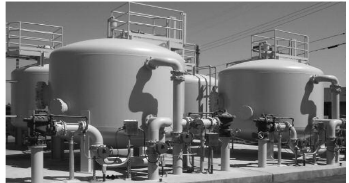
MetalEase-61 Installation in Elk Grove, California
